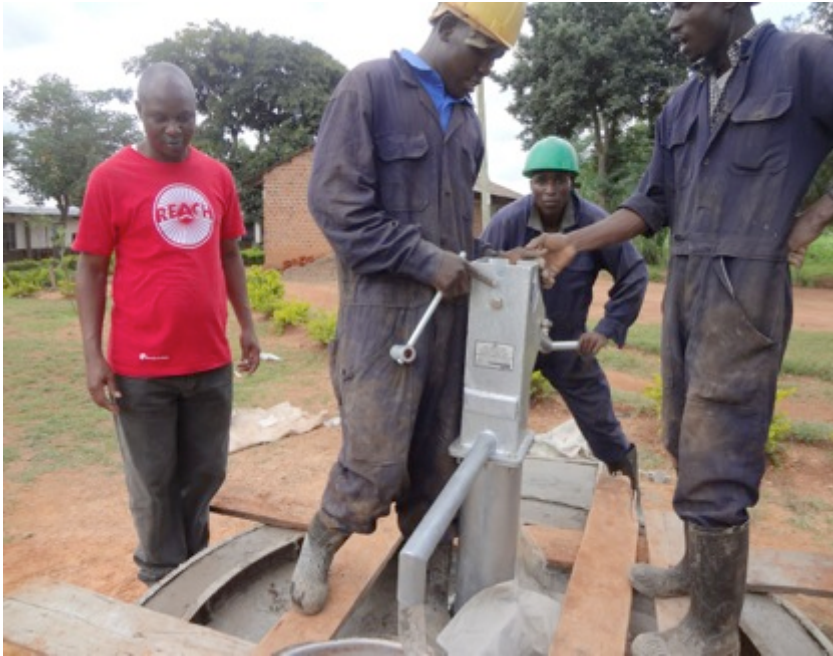
The drill team works to install the new hand pump.
